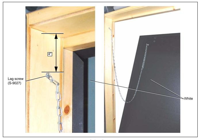
Figure 3H Safety Chain Installation
