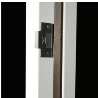
The Kerf Encapsulated Foam weatherstrip on the jamb is field replaceable.
