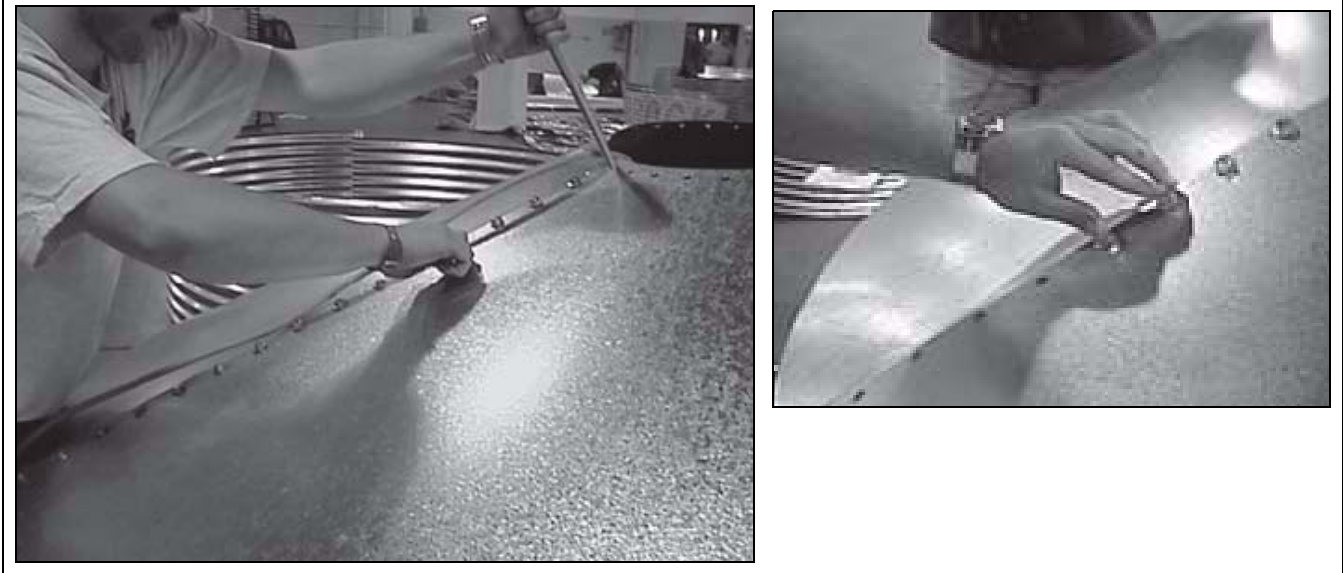
Figure 7B Lining Up Holes and Placing Bolts
